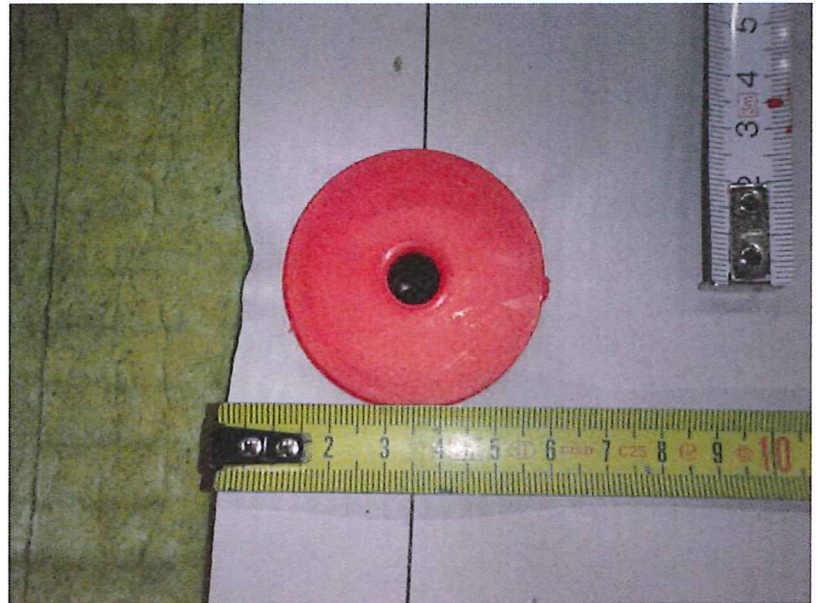
Foto 4 The distance from the fastening system to the edge of the roof waterproofing sheet.
